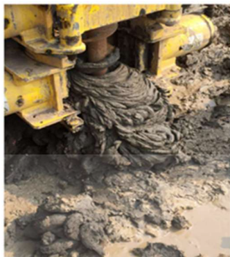
Fig. 2. Soft soil layer at the base of the waste dumpsite confirmed by the mudflow at the base Hoy et al. [2].
